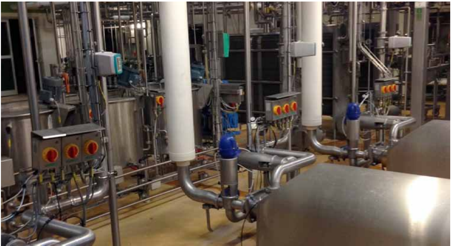
Stainless steel safety switches at Arla Foods
