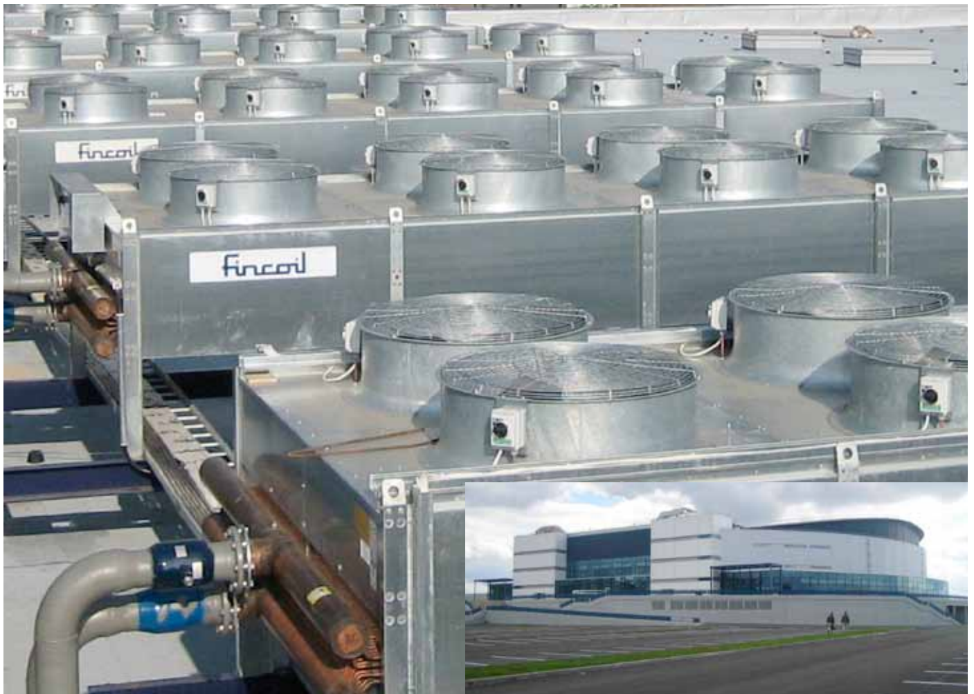
KATKO safety switches with ventilation machinery in Kazan Sports Arena, Russia
