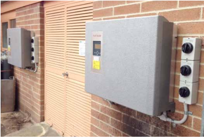
NEW KATKO DC isolators installed within a 30kW Solar System at Vines Golf Club (SA), Australia
