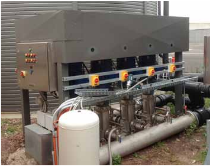
KATKO VSD EMC Isolators installed at Sydney International Airport, as part of two Santerno Multipump Systems for their Recycled Water Treatment Plant
